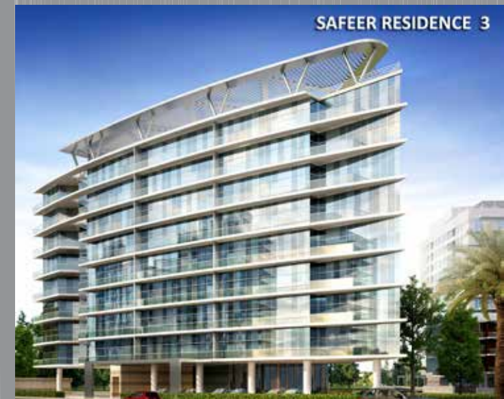
SAFEER RESIDENCE-3 Dubai Land Residence Complex
