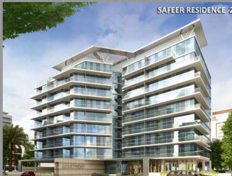
SAFEER RESIDENCE-2 Dubai Land Residence Complex
