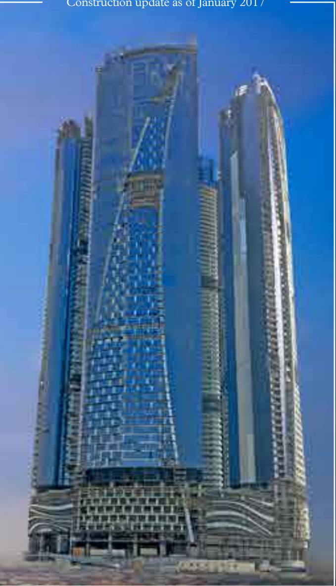
Construction update as of January 2017
